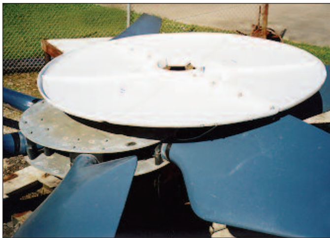
Typical Seal Disc Prior to Installation Fig. 13
