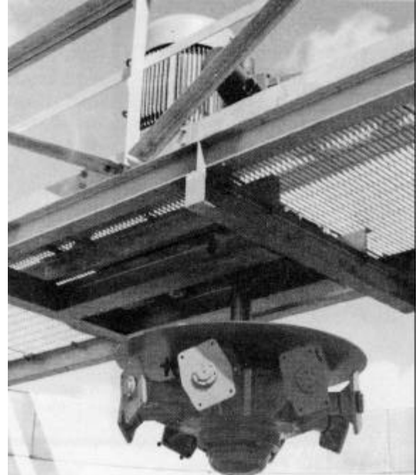
Figure 3 Electrically Operated Variable Pitch Fan
