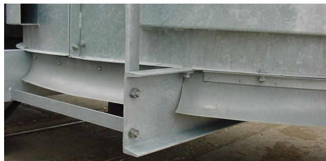
▲ Figure 9. An inlet bell can increase the total airflow in an air-cooled heat exchanger by 2–3%.
