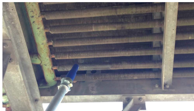
▲ Figure 12. Dry cleaning is one of the most effective methods of cleaning the airside of tubes and is the least likely to damage the finned tubes.
