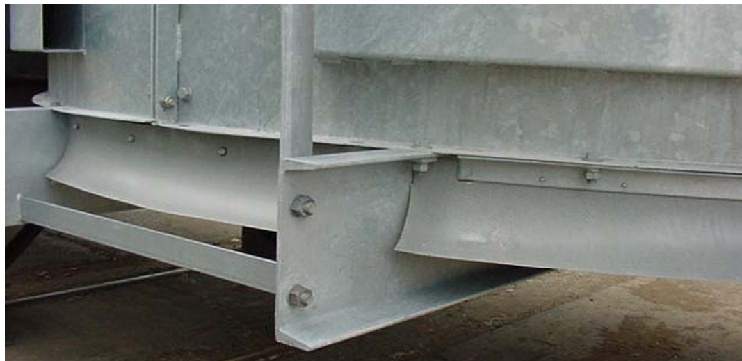
Figure 7. Typical ACHE inlet bell
